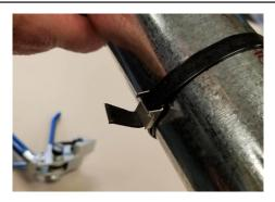
BEND CLIP WINGS DOWN TO SECURE STRAP
