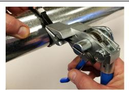
TIGHTEN UNTIL TIP OF TOOL PRESSES TIGHTLY AGAINST CLIP
