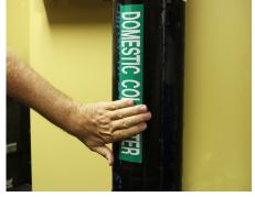
Align and lightly adhere one end of the marker to the pipe or insulation
