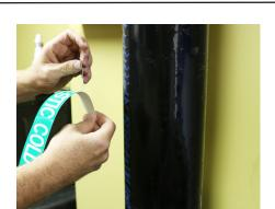
Smooth the marker from one side to the other using pressure to fully apply
