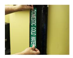
Apply arrow tape 360 around pipe, to include end of pipe marker
